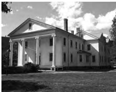
Historic Deep Energy Retrofit, Smith College
