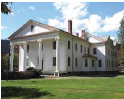
Historic Deep Energy Retrofit, Smith College
